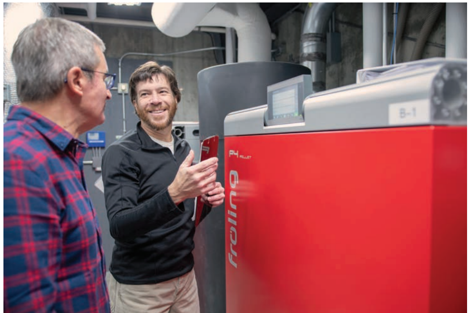
Dave Frank, co-founder of SunWood Biomass, and Mané Alves, founder of Vermont Artisan Coffee & Tea Company, look over a wood pellet boiler system installed at the coffee company's Route 100 facility in Waterbury. Photo credit: Erica Houskeeper
